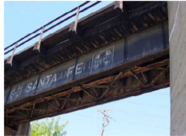
Steel Plate Girder
