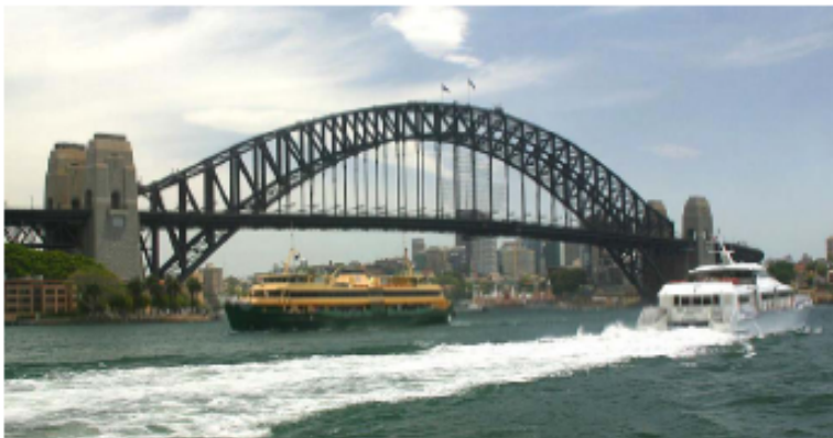
Sydney Harbor Bridge (1938) Sydney, Australia parabolic arch 503 m span
