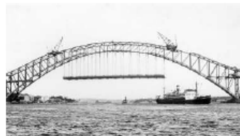
Construction of Sydney Harbor Bridge
