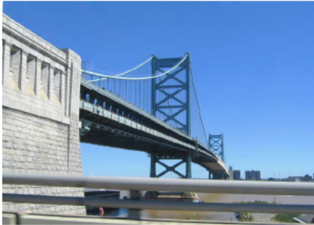
Anchor of a suspension bridge
