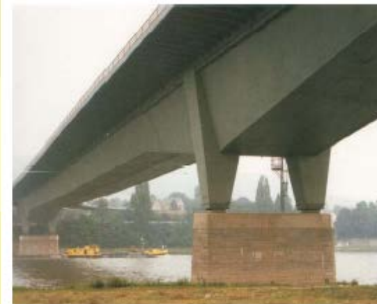
Steel Box Girder Bridge
