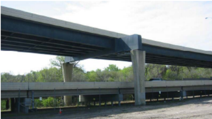
Upper: Steel Plate Girder Bridge Lower: Prestressed Concrete I-Girder Bridge
