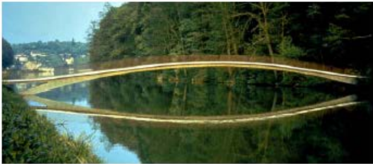
Enz Bridge (1961) Mülacker, Germany 46 m span Concrete arch
